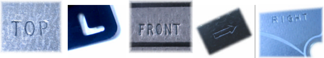
Some of the common gasket markings that indicate special fitting orientation
